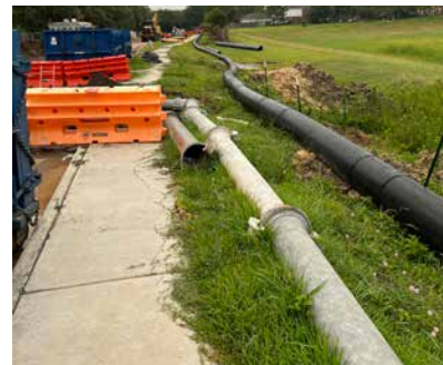
Bypass lines, 180' metal (L) & 800' HDPE
