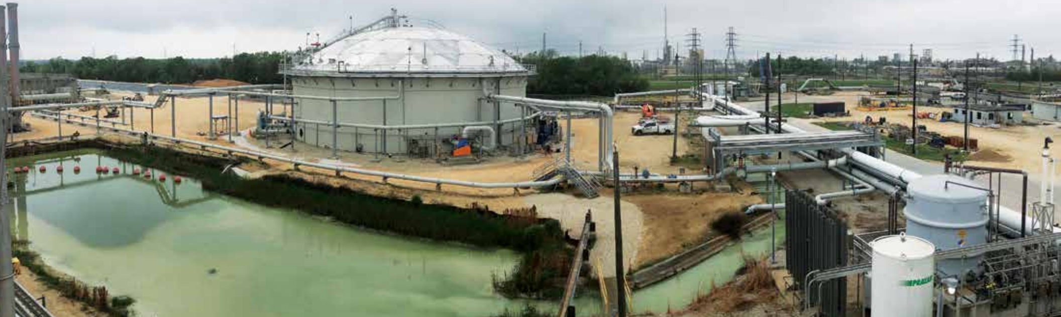
The Bayport improvement project is making significant progress. Pictured is the new T-2005 First Step Aeration Tank, along with the associated piping and recirculation system equipment.
