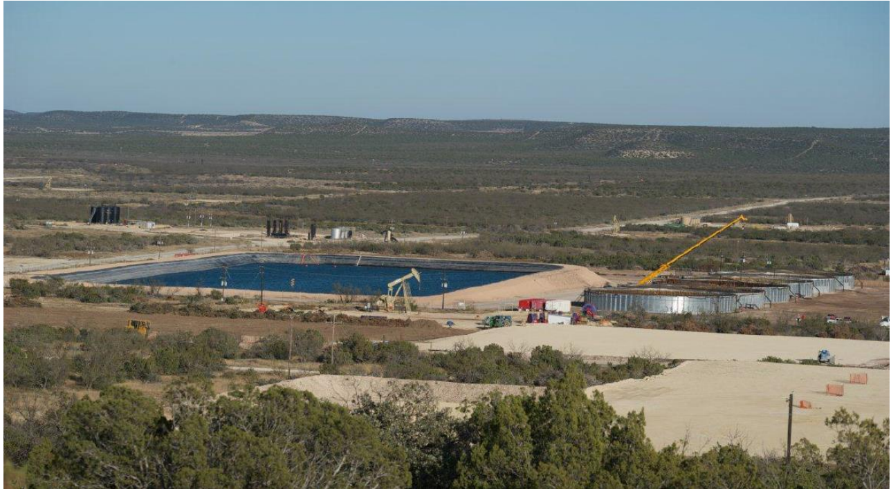
Figure 5.2 Brackish Water Pit and Holding Tanks in Irion County, Texas
