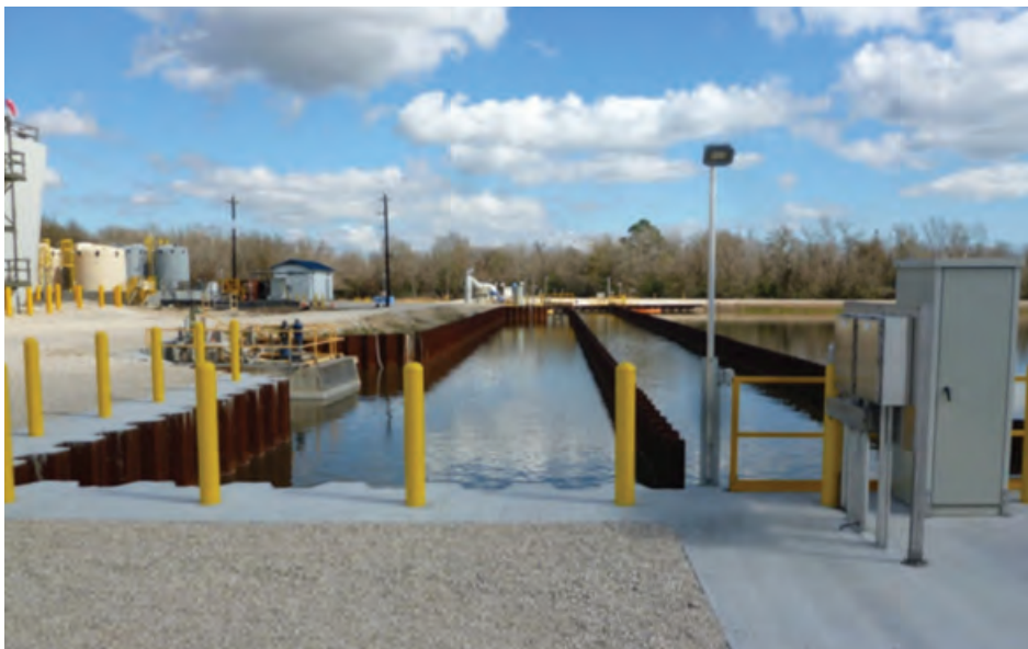
The pond with baffling installed to provide appropriate retention time for the new disinfection system.
