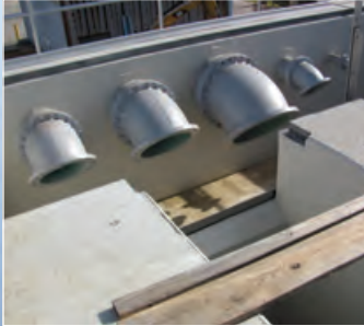
Termination of the four force mains coming into the Blackhawk facility
