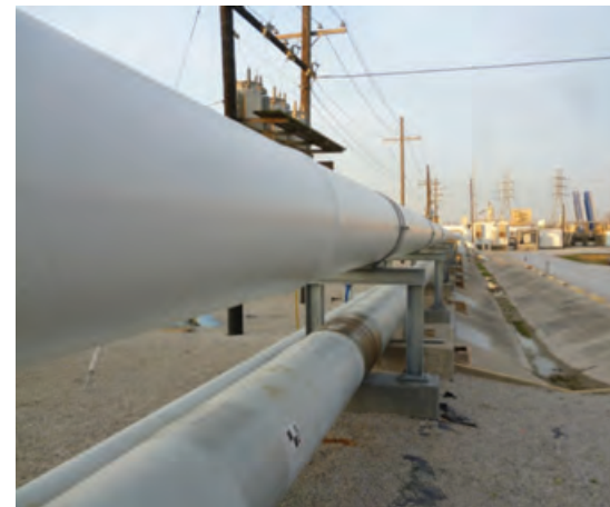
Part of the lift station improvements included replacement of the existing line with a larger 42-inch line connecting the station with first-step treatment tanks.
