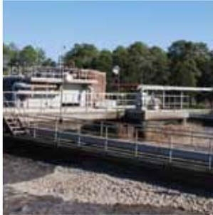
Wastewater is transported by pipeline to the facility, where it undergoes primary, secondary and advanced treatment, including filtering through sand and charcoal and disinfection by ultraviolet (UV) light, prior to discharge into Clear Creek.
